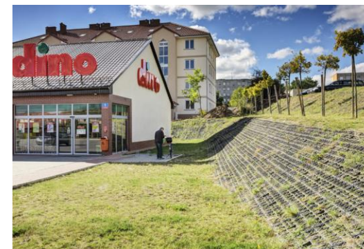
Escarpment reinforcement by a store, Świebodzin
