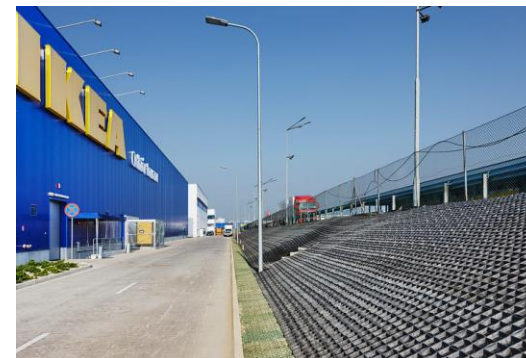
Embankment reinforcement by the IKEA store, Poznań
